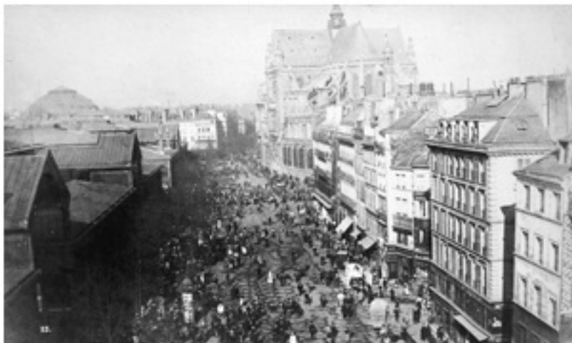
Les Halles and Saint-Eustache, late nineteenth century
